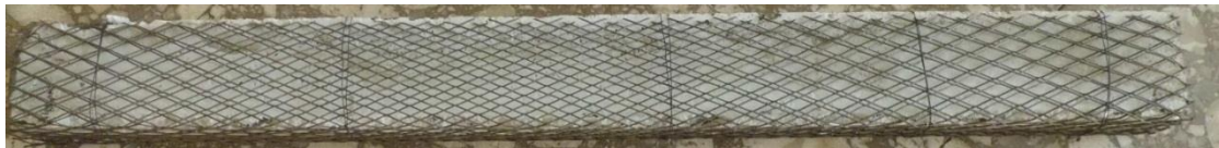
Repairing of beam b6 by two layers U shape expanded steel mesh.
